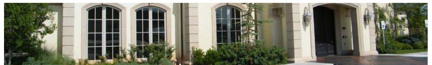
The building has a French Provincial design with a stucco and cast stone exterior facade.
